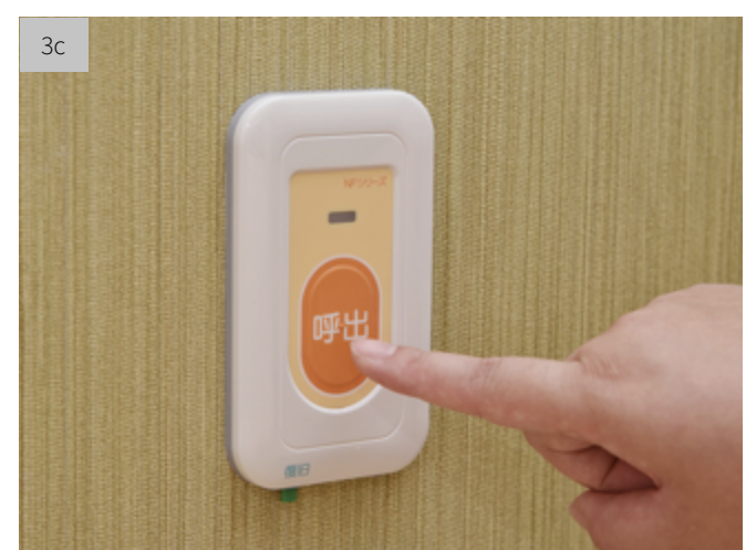
Figure 3a: View of Yuimarl Fuku Figure 3b: Interior of an individual unit Figure 3c: Emergency bells are fitted in the room
