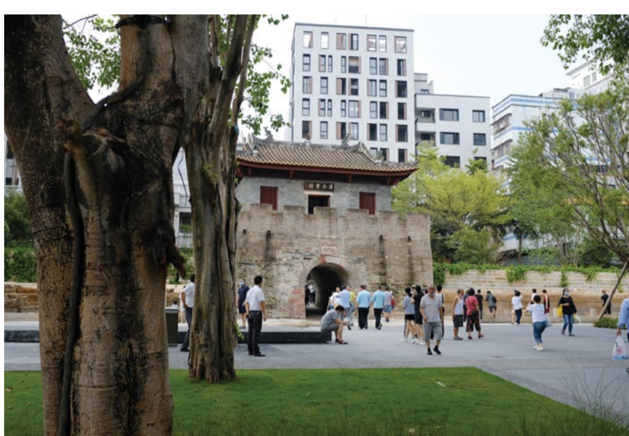
Retaining cultural personality is a key consideration in the rejuvenation of areas in Nantou Ancient City. Source: Urban Planning & Design Institute of Shenzhen
