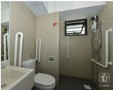
Wheelchair accessible bathrooms fitted with grab bars.
