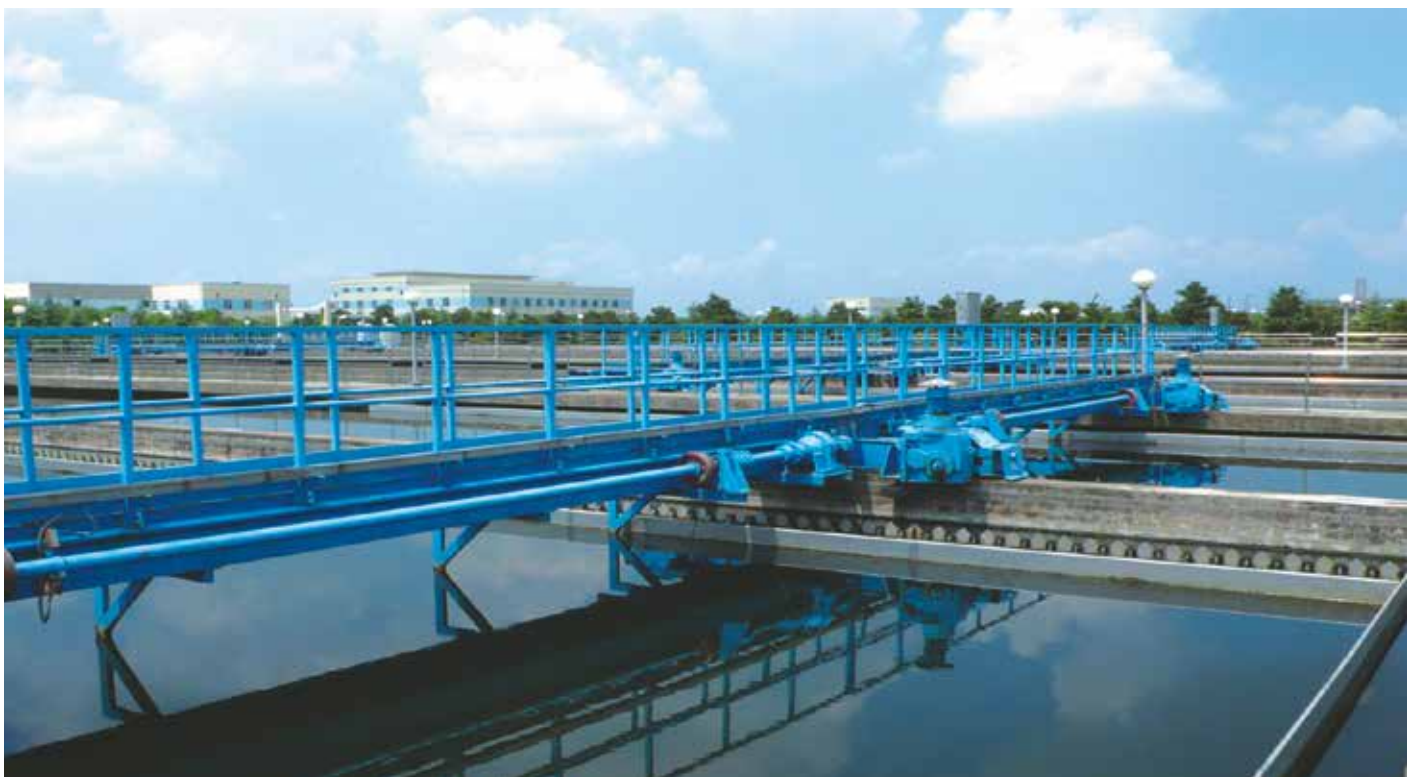
Waste water treatment plant
