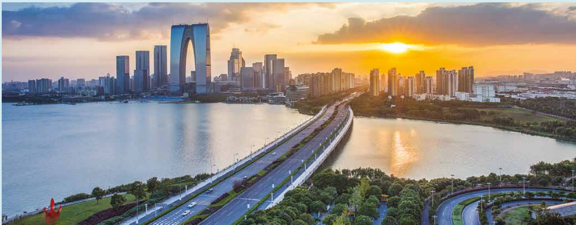
Jinji Lake Bridge
