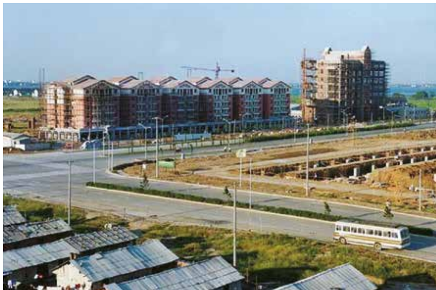
Xindu Plaza (Depicted under construction and after completion)
