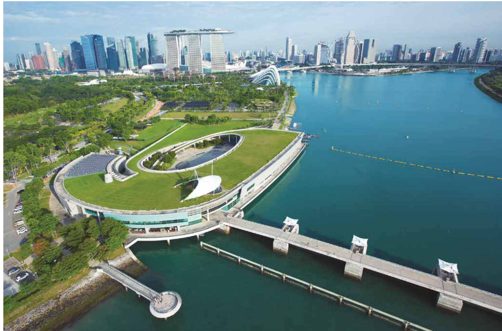
Bottom The Marina Barrage is a multi-use space that fulfils functions of flood control, urban water catchment and public recreation. Source: PUB, Singapore's National Water Agency
