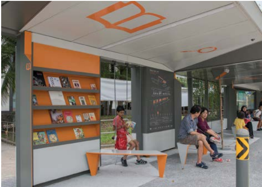
Project bus stop in Jurong East designed by DP Architects where commuters can enjoy free Wi-Fi, charge their mobile phones, download e-books and sit on a swing.
