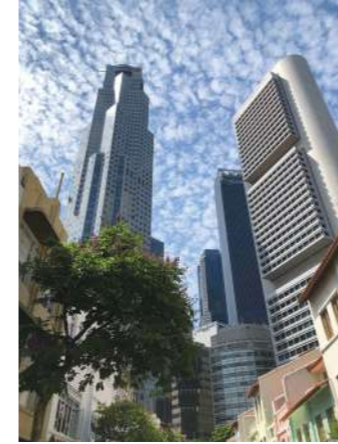
Roofscape of UOB Plaza (left in image) and OCBC Centre (right in image). Source: Nikhil Soni/Pexel
