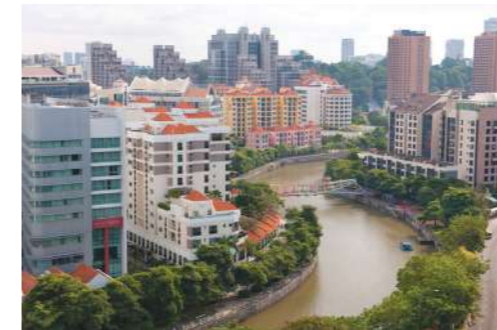
Top: Redeveloped sites featuring this mixed height typology along the river include The Quayside and River Place. Source: URA Right: Schematic section showing the maximum 4- and 10-storey building height typology at Robertson Quay. Source: URA
