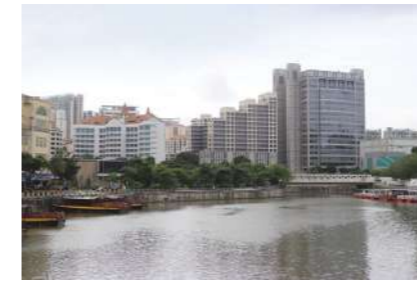
The stepped building height at UE Square, in response to the developments along the river. Source: Victoria See, 2022
