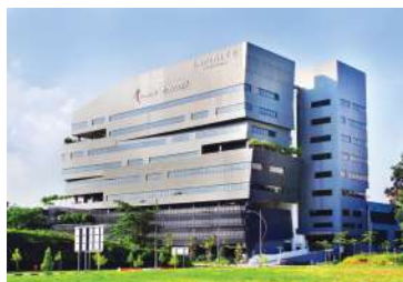
Infinite Studios. Source: DCA Architects
