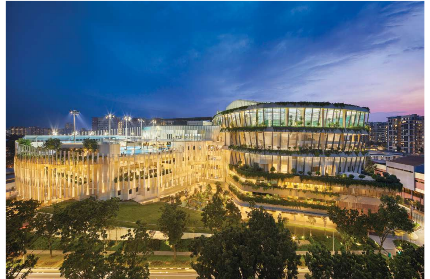
The 45°-sloping window detail reduces the glare from Heartbeat@Bedok’s internal lighting onto the surrounding blocks at night. Source: ONG&ONG
