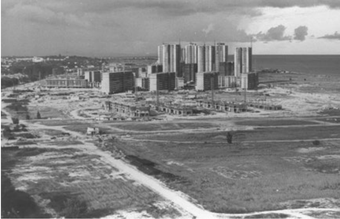
Housing and Development Board (HDB) flats under construction at Marine Parade in 1973. (Marine Parade Community Centre Collection, courtesy of National Archives of Singapore)
