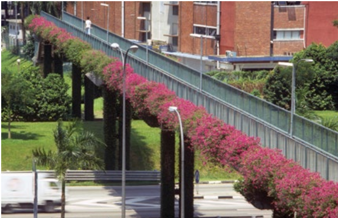
Overhead bridge in Telok Blangah, 1990. Mr Wong Yew Kwan, Singapore's first Commissioner of Parks, proposed the installation of troughs along overhead bridges to house flowering shrubs like Bougainvillea . (Ministry of Information and the Arts Collection, courtesy of National Archives of Singapore)
