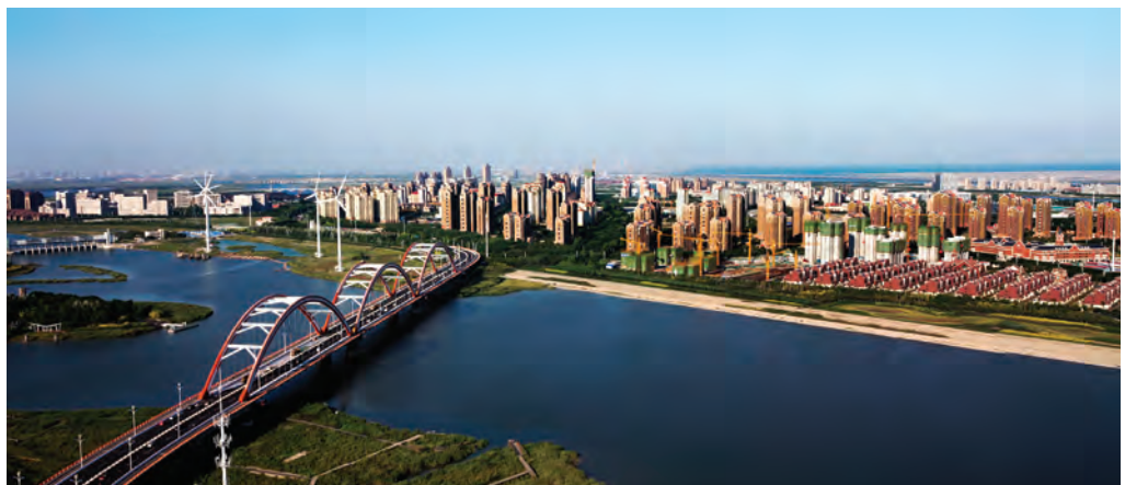
After (2015). Photo credit: Ministry of National Development
