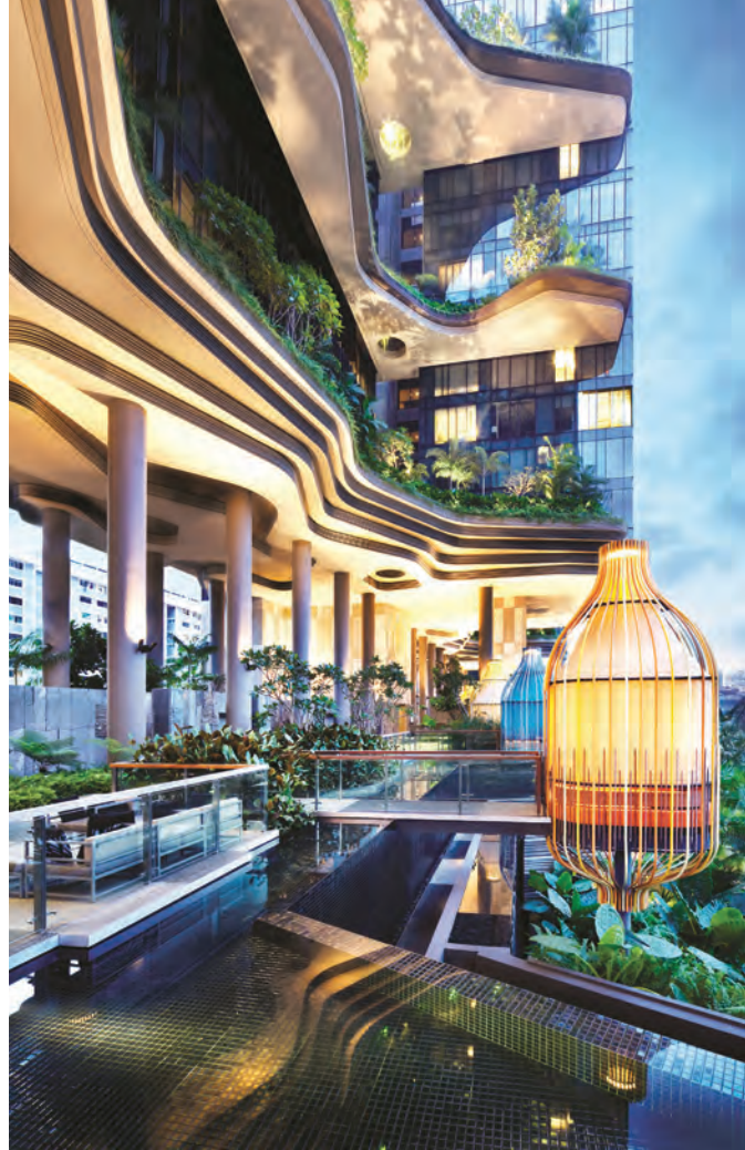
PARKROYAL on Pickering, a BCA Green Mark Platinum Non-Residential Building. Photo credit: PARKROYAL on Pickering
