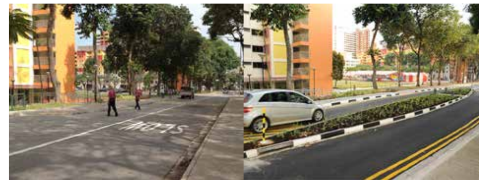
Before and after the addition of an “Eye-land” in the middle of the road.
