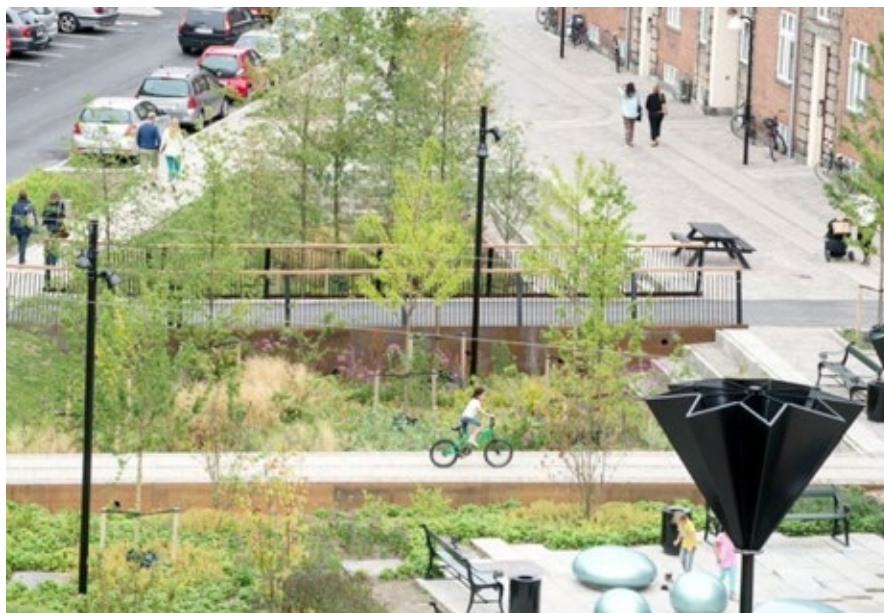
Figure 4: Tåsinge Plads: Water from the street flows into flowerbeds during heavy rains, while sculptures collect water to nourish plants, creating capacity in the drains to prevent flooding and damage.
