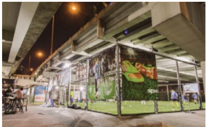
Offside at Thomson Flyover. Source: Urban Redevelopment Authority
