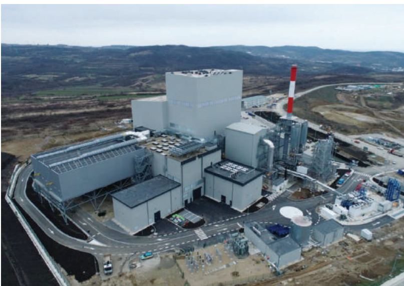
In February 2023, the facility started the production of electricity and heat from waste. Image: Beo Cista Energija
