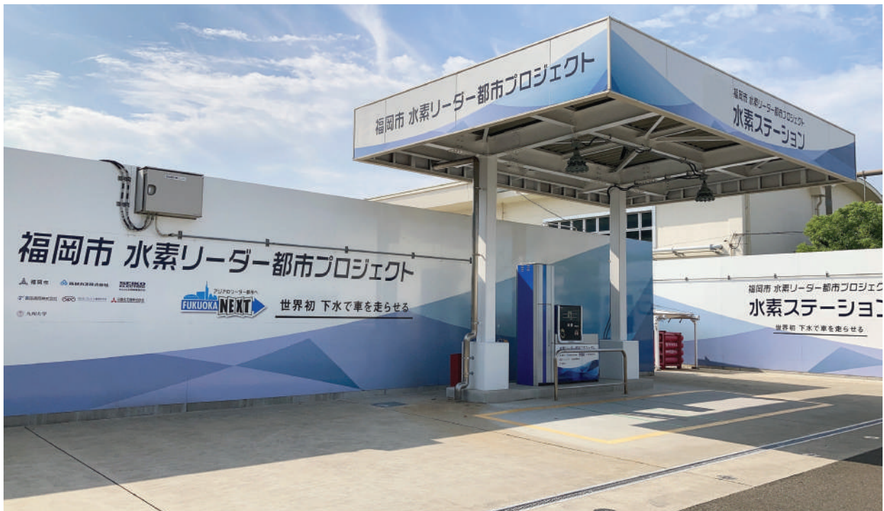
| A world-first hydrogen station that produces hydrogen from sewage. Image: Fukuoka City
