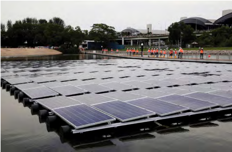
One out of ten floating solar systems being tested at Tengoh Reservoir. Image: TODAY
