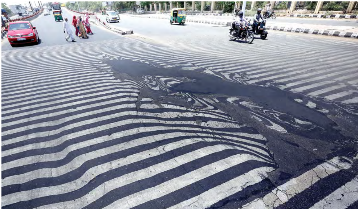
Road markings appear distorted as the asphalt starts to melt due to the high temperature in New Delhi, India. In June 2019, temperatures touched 48°C, the hottest June day in the Indian capital on record. Image: Harish Tyagi / EPA
