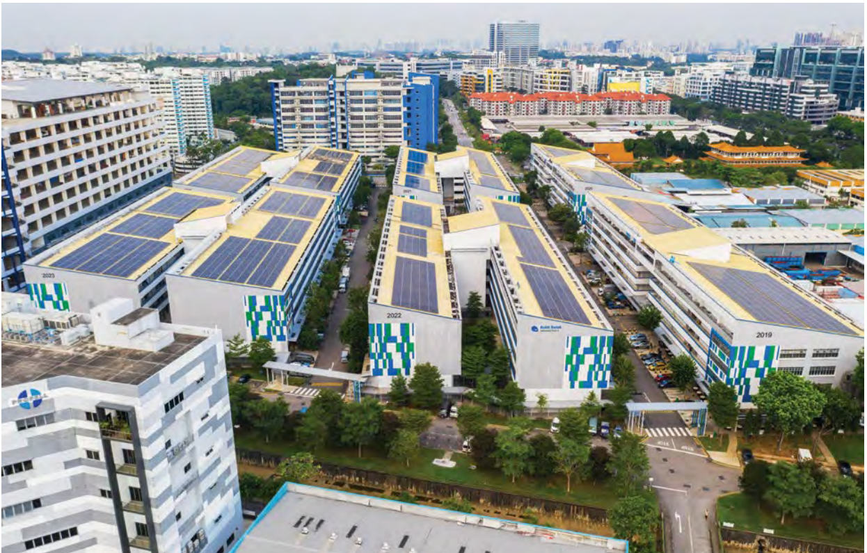
Solar panels on the roof of factories in Singapore. By 2030, Singapore will ramp up its solar capacity by more than seven times from current levels. Image: Aerial / Alamy Stock Photo
