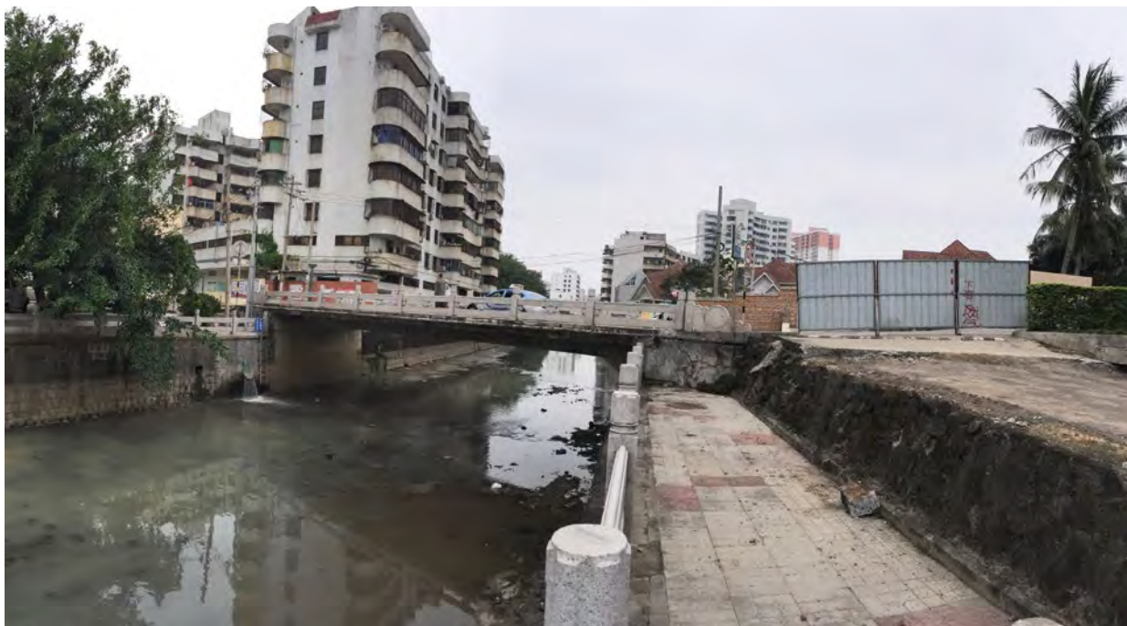
Before the “grey-to-green” project, Meishe River was a lifeless, concretised waterway. Image: Turenscape
