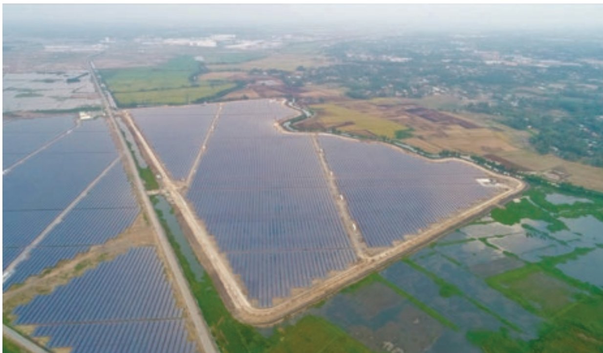
A solar array that Standard Chartered financed in Vietnam. Image: Asian Development Bank
