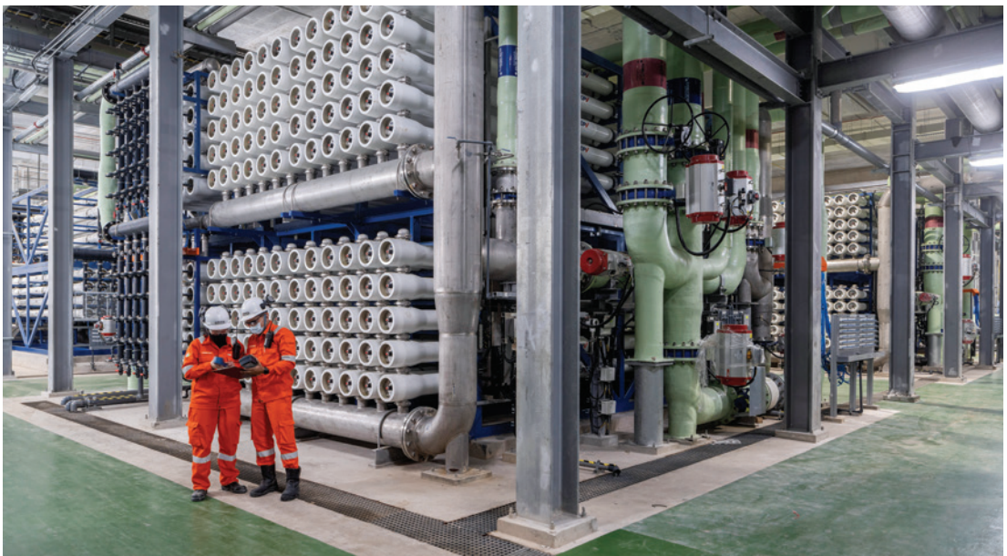
Aerial shot of Marina East Desalination Plant (MEDP) and reverse osmosis system. Image: Keppel Infrastructure
