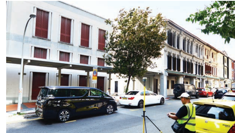
The substation (left of picture) along Tras Street, with its façade carefully designed to fit into the surrounding area.
