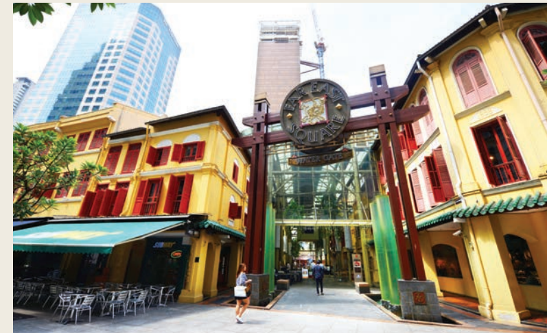
Restored shophouses that are part of Far East Square, one portion of the China Square Development.
