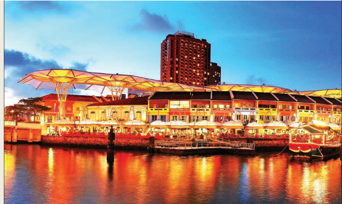
Clarke Quay's unique and iconic umbrella structure. Courtesy of Singapore Tourism Board.
