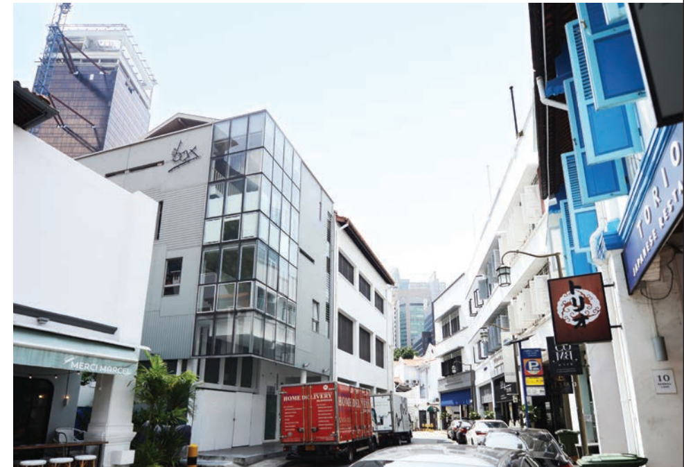
An in-fill building added to a row of conserved shophouses, built in accordance with envelope control guidelines.
