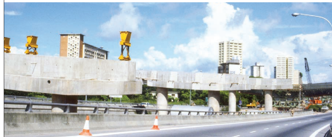
Construction of the East Coast Parkway (ECP).
