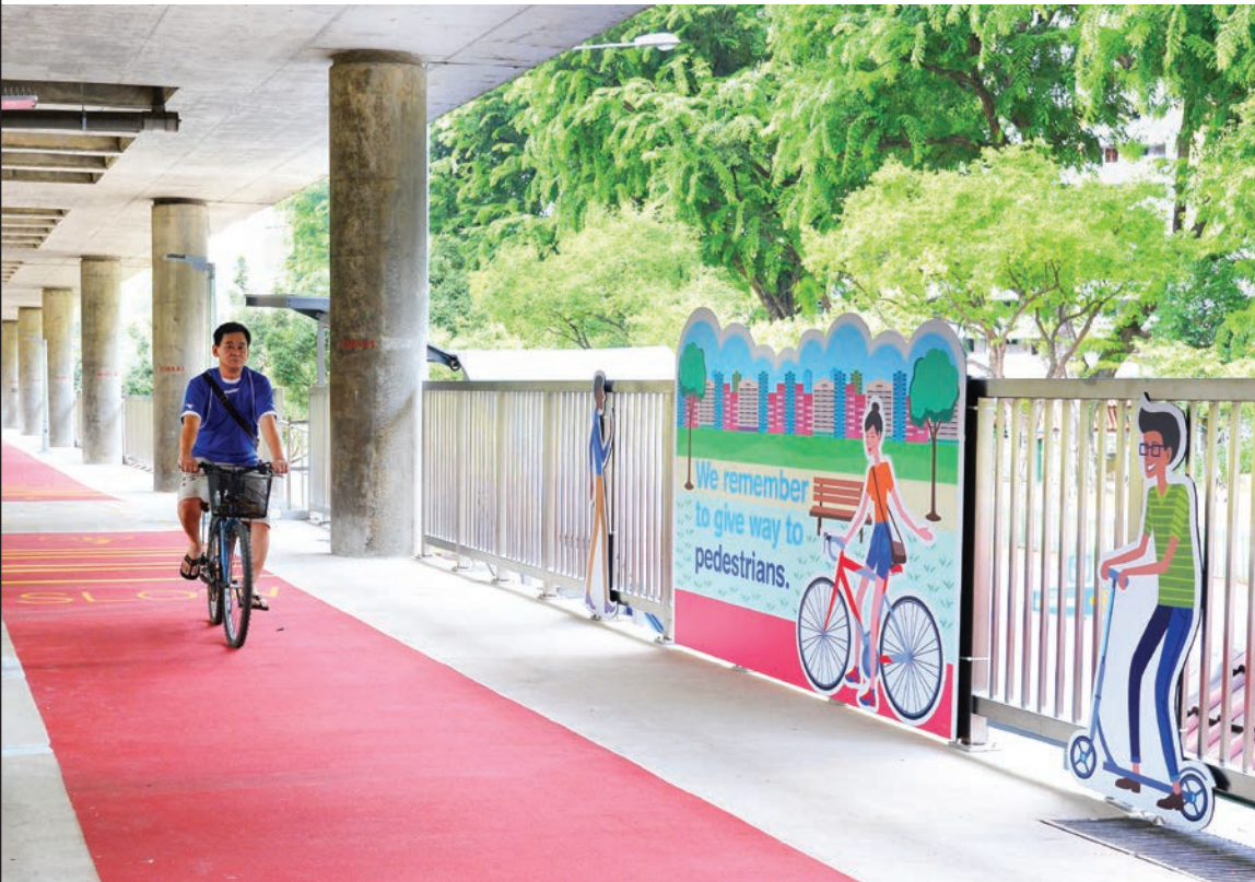
Ang Mo Kio Linear Park under the viaduct of the North South Line. Photo courtesy of Land Transport Authority.
