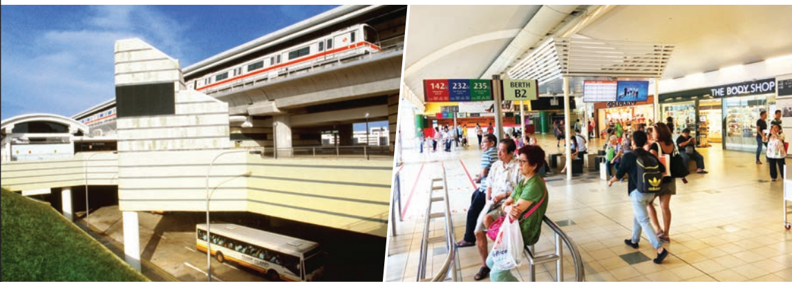
Woodlands MRT station above the bus interchange (left) and Toa Payoh Integrated Transport Hub (right).
