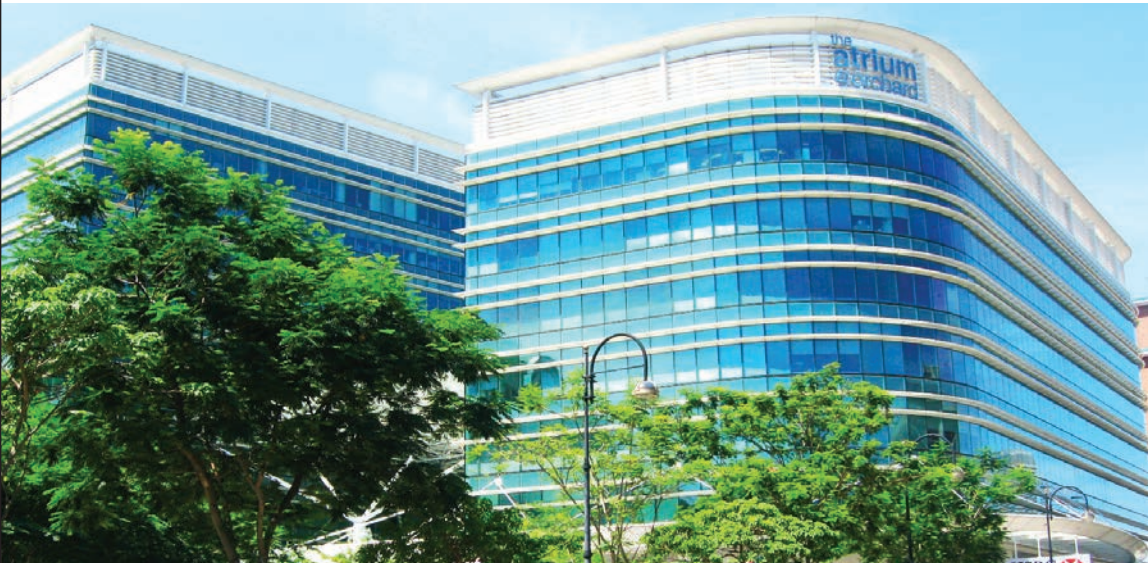
The Atrium@Orchard built above the Dhoby Ghaut NEL station.
