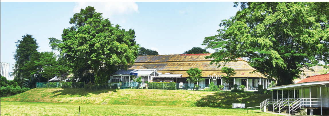
Dempsey Cluster, Tanglin Village. Image courtesy of the Singapore Land Authority.
