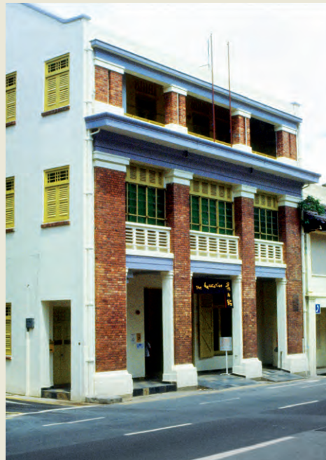
Facade of The Substation at Armenian Street (1991).
