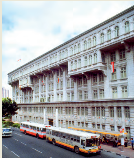
Old Hill Street Police Station (1982).
